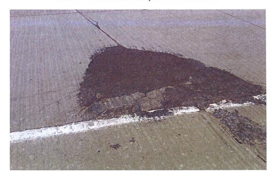
Photo 1 – Photo of bituminous patch on Lookout Drive.
